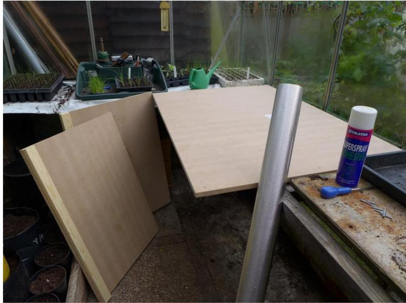
The reflective Diamond Mylar material was stuck on with spray adhesive.
